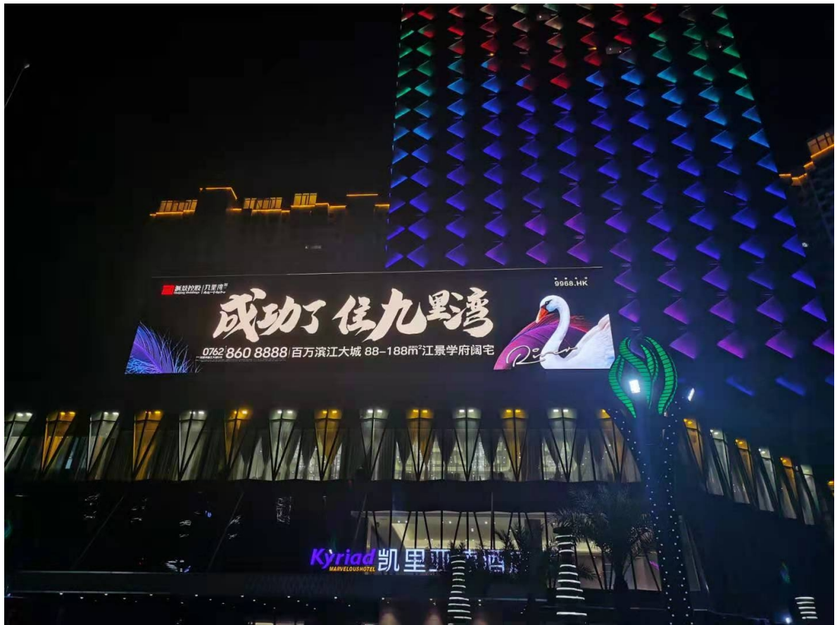
LED 三面翻显示屏实景拍摄
